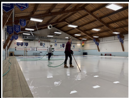
We altered our hot water system for improved water quality and clarity.
